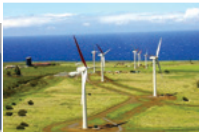
Wind farm at Hawi, Hawai'i Island
