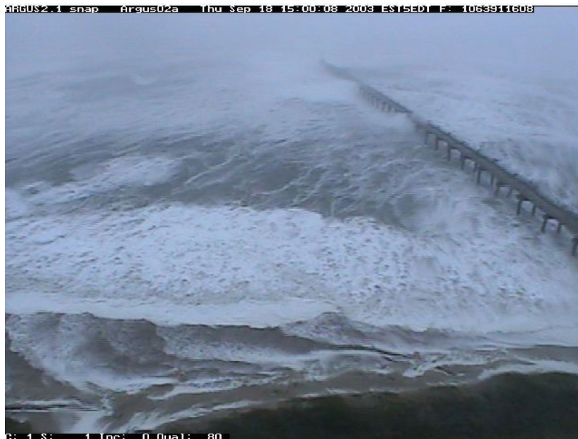
Figure II.B.1. Waves overtop the 8 m tall research pier at Duck, NC, on September 18, 2003, during Hurricane Isabel. Because of the permanent coastal observing system maintained at Duck, continual records of bottom boundary layer currents are available during major storms. However, highly energetic, episodic conditions are generally under-sampled worldwide. Photo courtesy of the US Army Corps Field Research Facility.
