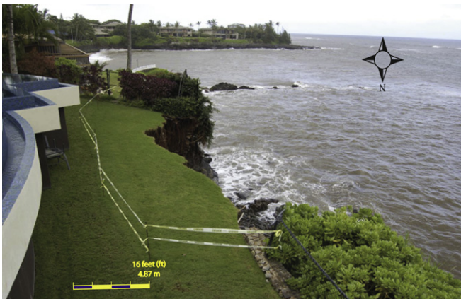
Fig. 6. Setbacks must account for catastrophic cliff failure.
