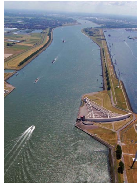
The Netherlands has traditionally defended itself against the sea with concrete and metal structures, such as the storm-surge barrier Maeslantkering, near Rotterdam.
