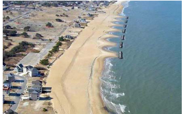
Offshore breakwaters can keep sand onshore, reducing the rate of shoreline erosion.
