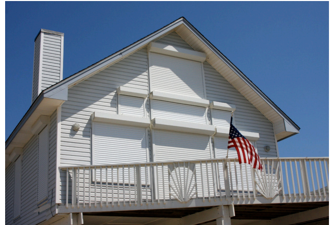
Hurricane shutters can be added to existing structures to reduce the damage caused by wind and water.
